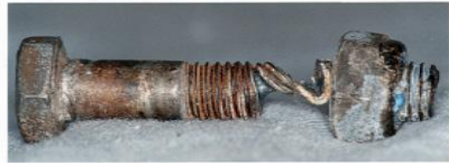
Lower bolt failure
